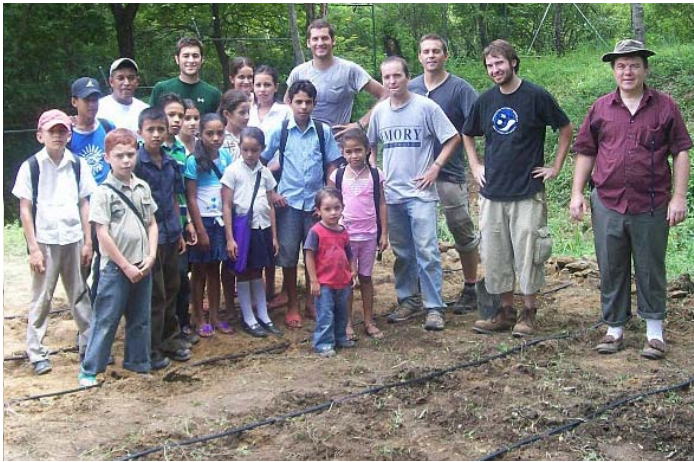
Six members of the EOS team stand proudly with the students of a school in Palmar Sur, Nicaragua after working together to install a drip irrigation system on their school grounds. This system will be used to teach students about agriculture and the importance of water conservation while introducing this technology to an entire village.
